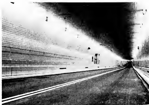
View of the Tunnel interior.
